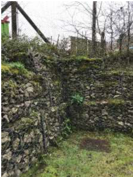
Plate 3 (Gabion Wall Reinforcement)
